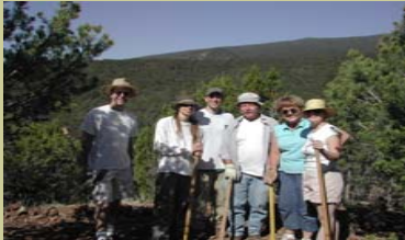
SMNHC Volunteers constructing a new trail.
